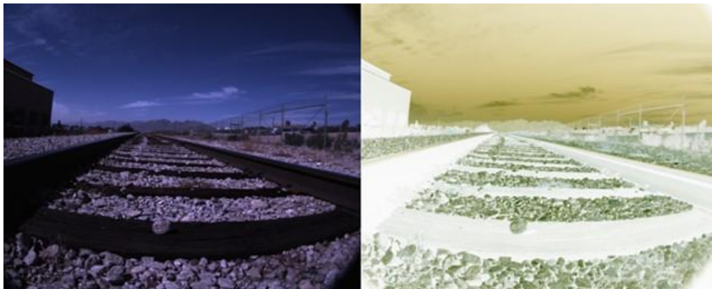
Figure 45 Rail images. (a) Rails in original condition. (b) Inverted binary image.
