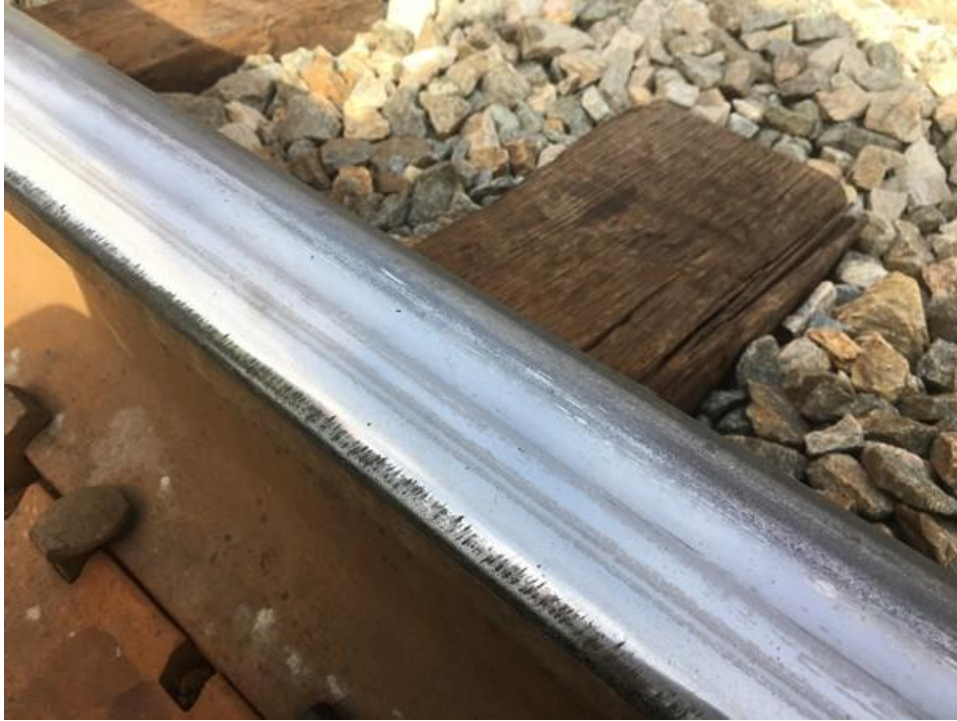
Figure 5-11: A field survey of the mainline track shows evidence of TORFM on the outside of the rail.
