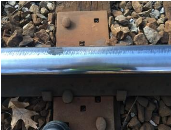
Figure 5-18: A patch of dried TORFM can be seen on the field side of the rail.
