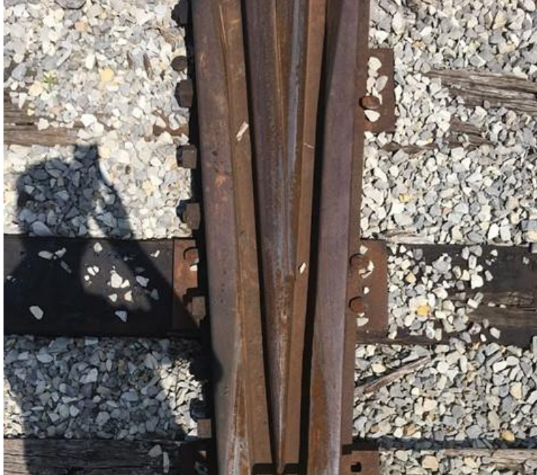
Figure 5-8: Example of a switch frog
