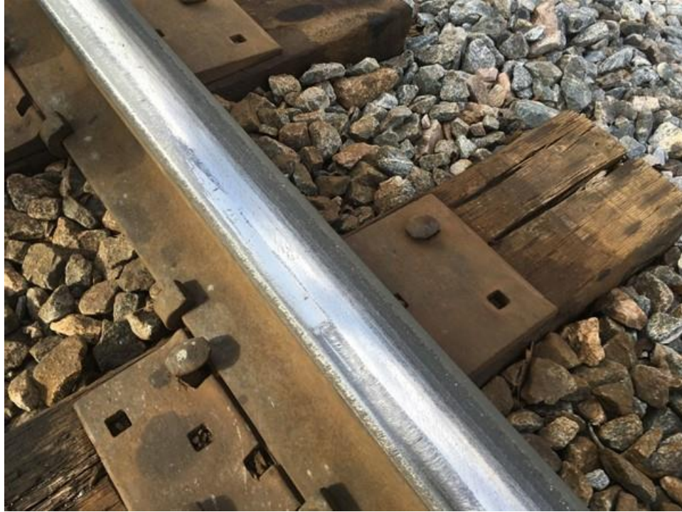
Figure 6-7: Non-uniform, "patchy" distribution of TORFM on the top-of-rail surface in a sharp curve
