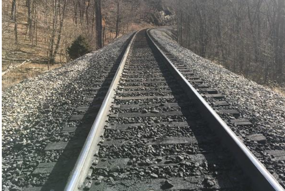
Figure 5-44: TORFM patches moving down track from a TOR applicator caused by the coherent phase of the train wheels
