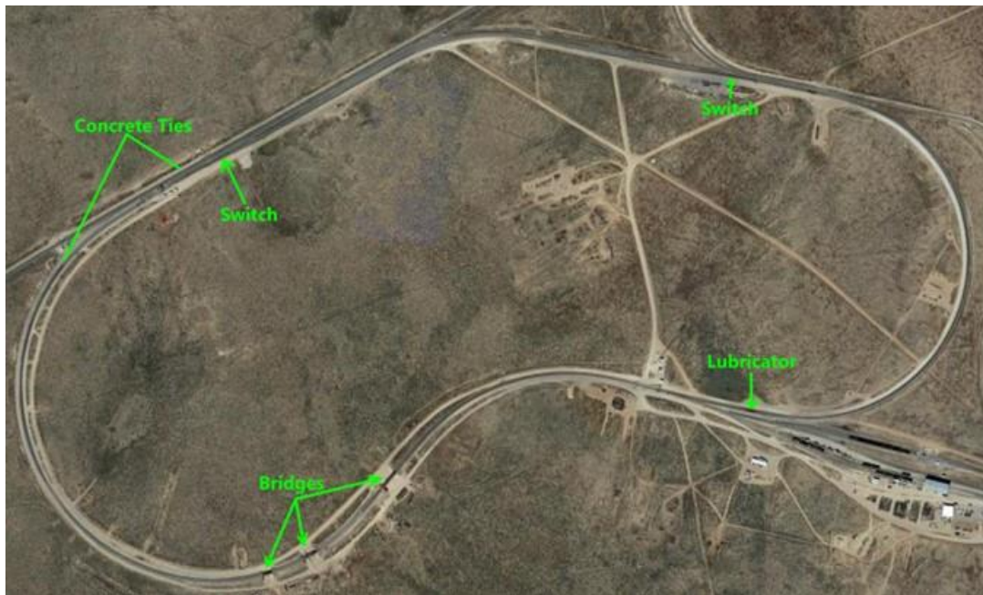
Figure 2-7: Additional elements found on the HTL such as switches, bridges, concrete ties, and a lubricator
