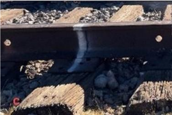
Welding defect: 0.3 in * 0.3 in. Location: 1.9 inches below the surface
