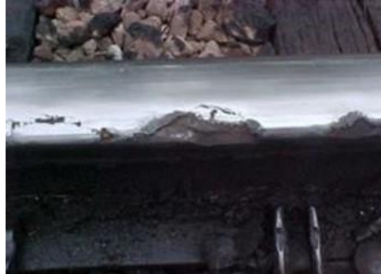
Side shells corrosion
