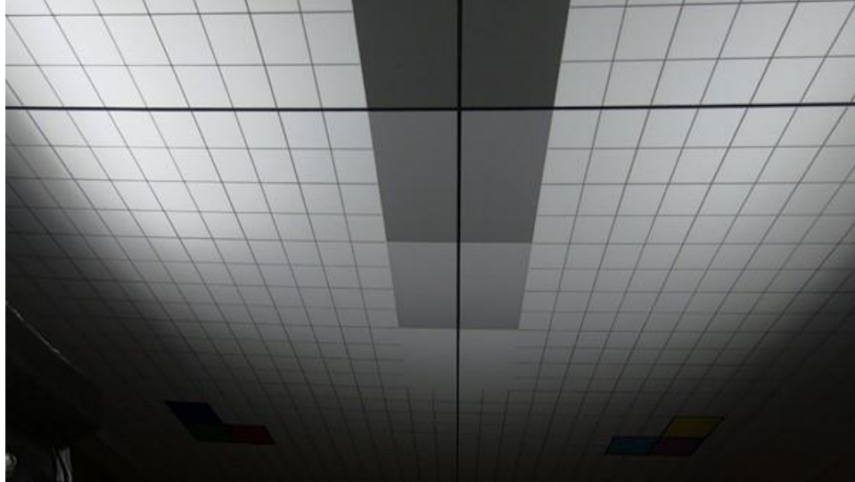
Figure 0-3: Side camera view showing the inability of the original lighting system to illuminate the outer regions of the FOV
