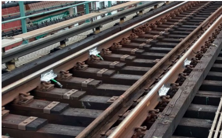
Figure 10 ISI L/V measurement system located north of 103rd street station (NYCTA).
