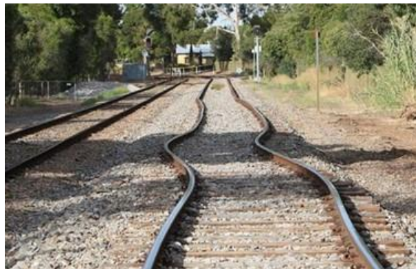
Figure 3 Buckling of tracks in lateral direction (Knapton 2015)
