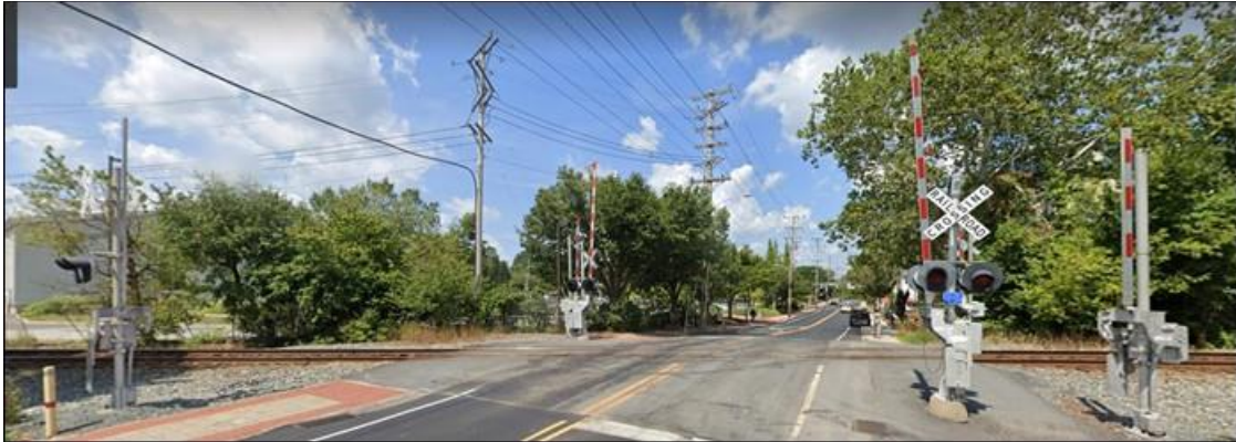
Figure 1: Typical Highway-Rail Grade Crossing with Gates
